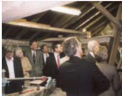
Surveyors check the timbers of the Whitechapel Bell Foundry.
